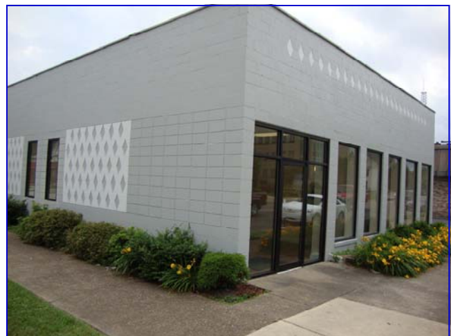
The new home for Marshall University CEGAS and its West Virginia Brownfields Assistance Center
