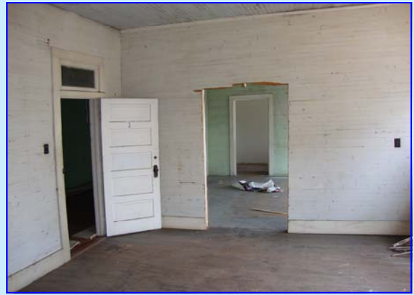
Interior View of Top Floor, Former Urlings Building
